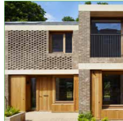
In this Morris & Company mews house in Sevenoaks waste storage integrated into the building frontage.
