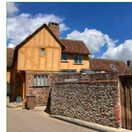
Barn St: Traditional flint and brick wall.
