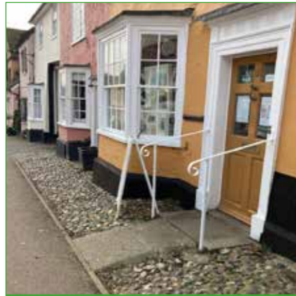
Edge and cobbled set-back demarcating ownership boundary.
