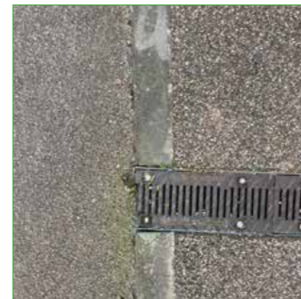
Bound gravel surfaces
