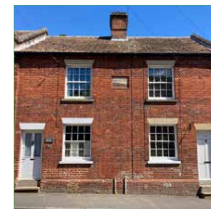
< The simple elevations of these homes display with a pleasing variety of complementary materials. Brick façade with contrasting pale opening surrounds and projecting horizontal band contrast with a simple off-white painted render.
