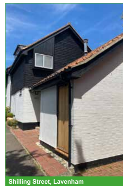
< Contemporary family home in Shilling Street with white painted brickwork and contrasting dark plinth detail and first floor weather boarding.
