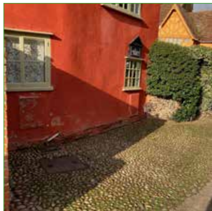
Edge and cobbled set-back demarcating ownership boundary.
