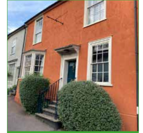
Stepped entrance with elegant handrail.
