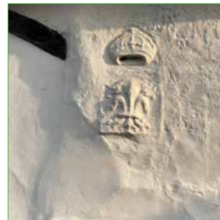
Plaster parqueting to facades
