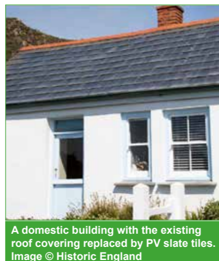
A solar PV array integrated into the slate roof. Image © Historic England
