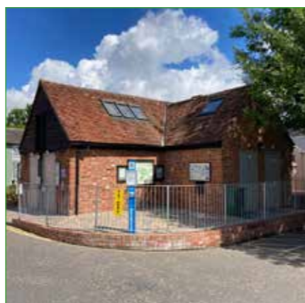
Public toilets, Cock Horse Inn Car Park
